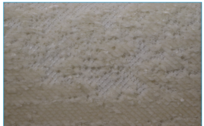
Severe scaling within feed spacers
